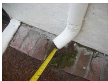
Picture represents several downspouts
